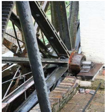
Daniels Mill waterwheel main bearing
