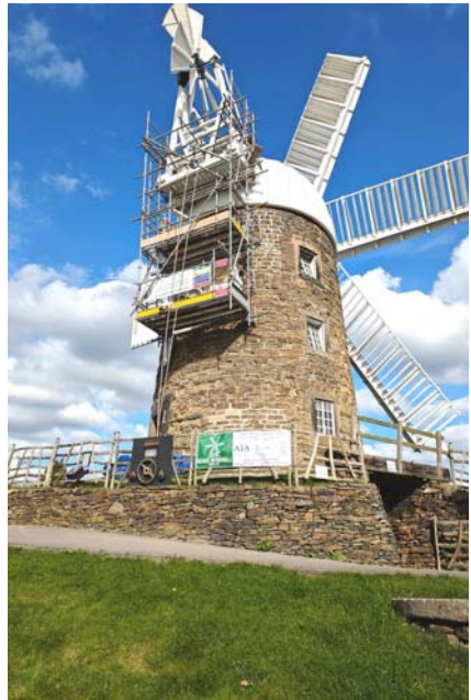
A long shot of Heage Windmill scaffolding (photo: Roger Hatchet)
